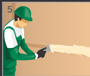
Finishing joint with SHERA jointing solution
